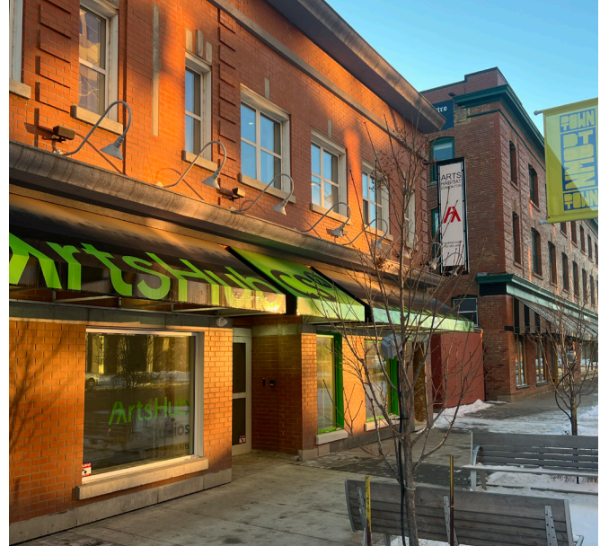
Completed Facade Construction at ArtsHub Creative Studios
